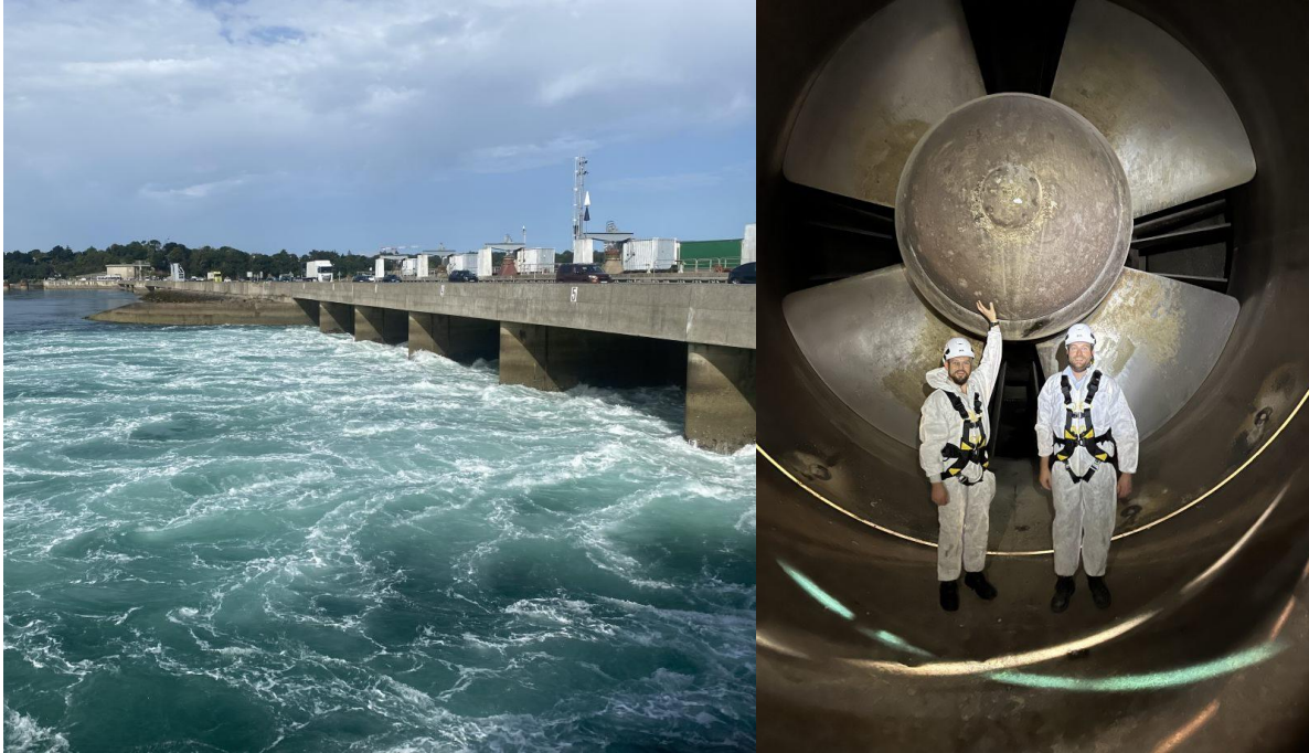
La Rance, St Malo, France, Operating since 1967 24 x 10 MW Units installed 500 GWh generation per year
