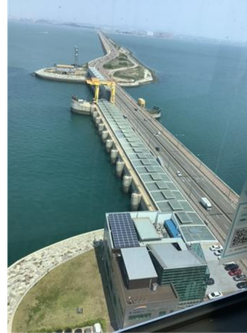
Sihwa - South Korea - K-Water Operating since 2014 10 x 25 MW Units installed 550 GWh generation per year
